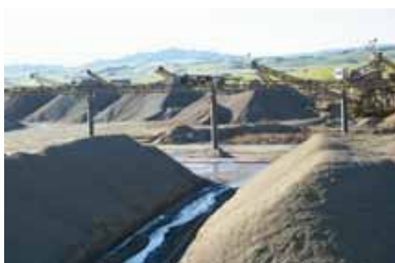
Figure 1: Paved Sand Stockpile Area – Tracy Aggregate Facility
